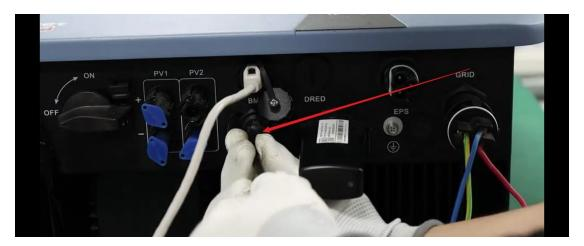
4. Connect the power cable of the energy meter to the grid.
